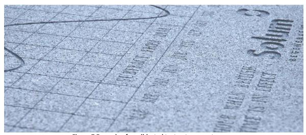
Figure 7 Example of sandblasted text onto concrete
